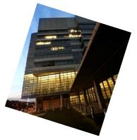
In strictest architectural parlance, a "curtainwall" is any non-load-bearing exterior wall that hangs, like a curtain, from the face of floor slabs, regardless of construction or cladding material. However, in common usage, the term curtainwall usually refers to aluminum-framed systems carrying glass, panels, louvers, or occasionally, granite or marble. Curtainwall supports only its own dead load.
