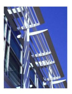
Exterior sun shades are used to block solar heat gain and increase Projection Factor (PF).
