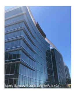
Early coordination between all exterior wall components and subcontractors is key to effective seismic movement accommodation.
