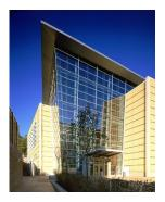
Can be stick or factory-assembled Field glazed using zone dams at frame corners
